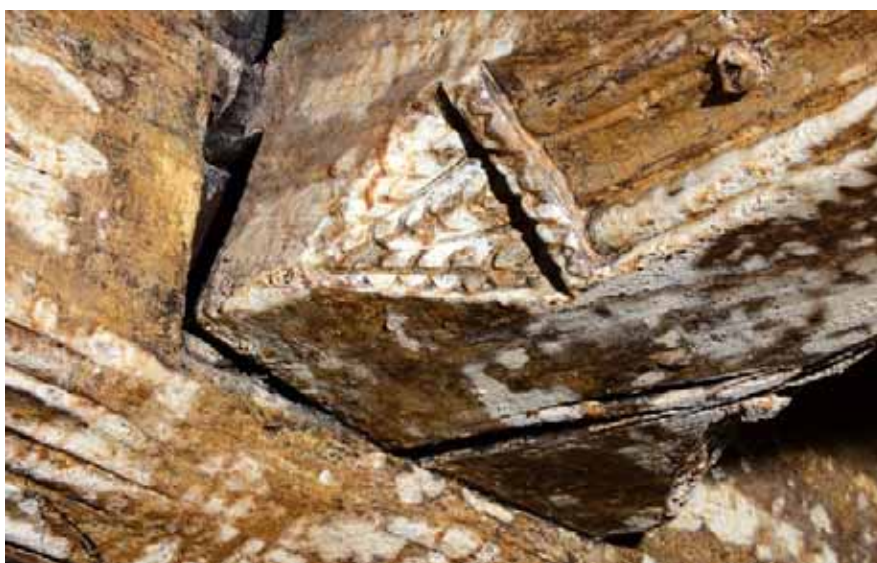
Figure 8: A particularly ornate chamfer stop previously undefined, but described here as a: Curved bar stop and incised. Source: © Historic England, Patricia Payne, image reference DP187931
